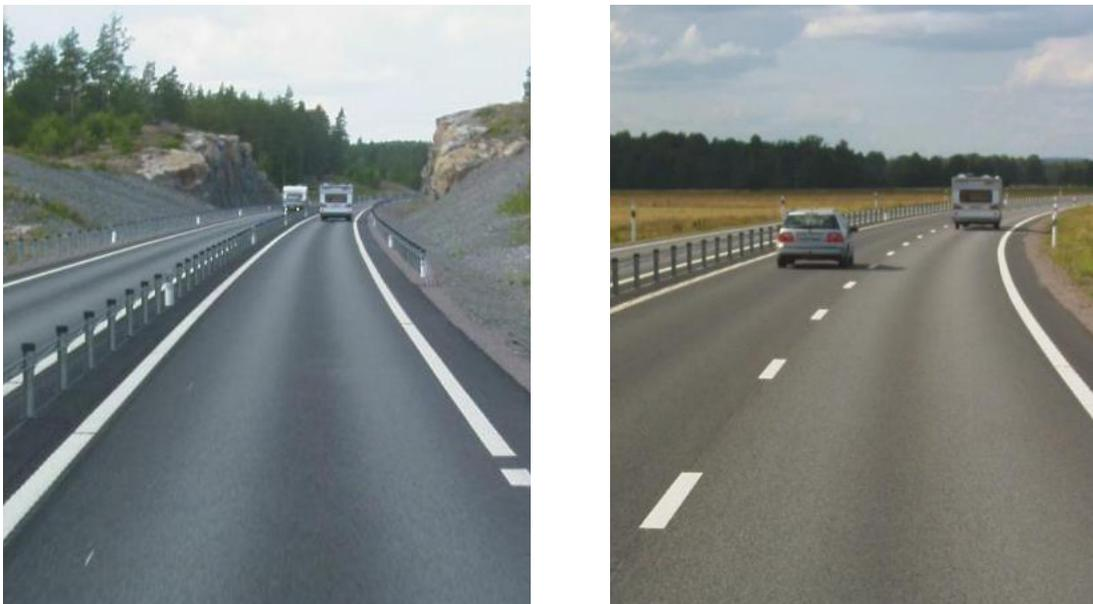
Figure 1: A narrow 2+1 road, width 9-10 m (left photo) and ordinary 2+1 road, width 13 m (right photo).
